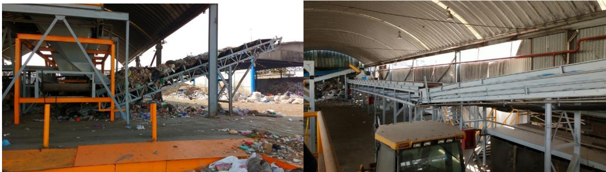
Fig. 4 San Juan de Aragón Sorting plant
