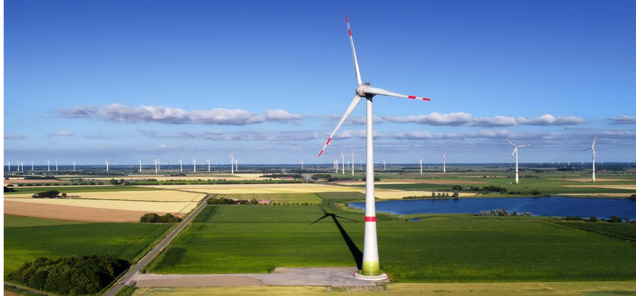
The rotor blades in wind farms turn majestically and seemingly at a constant speed in the airflow – here in a wind park near Emden. But the installation's output can double or halve within seconds.
