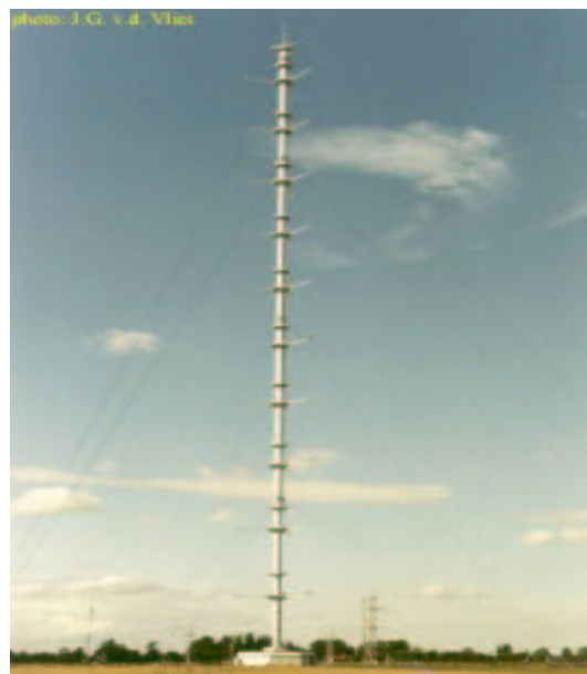
Figure 1: 200 meter high met mast in Cabouw, Netherland. The measurements are operated by the Royal Netherlands Meteorological Institute (KNMI)
