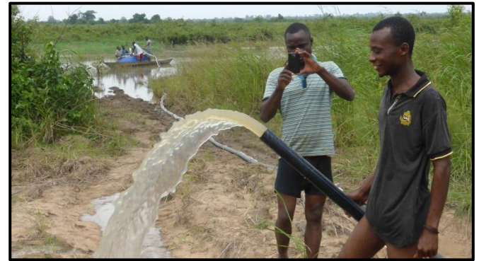
2.5 kW field irrigation system using PV Solar and a surface water pump (Aveyime, Volta)
