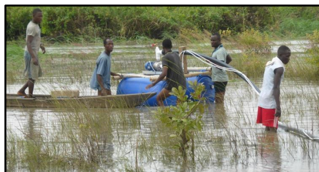
Pilot Project: Surface water irrigation system with surface pump on floating island (Aveyime, Volta)
