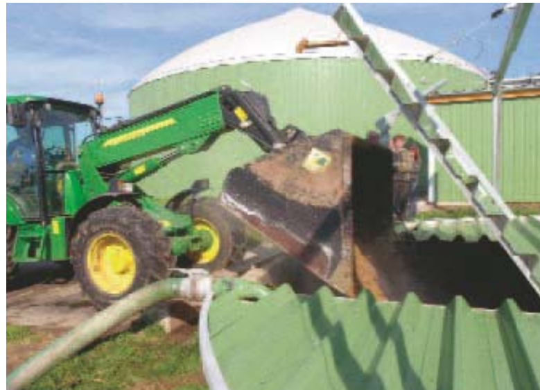
Brandenburg's most modern biogas plant in Pirnow
