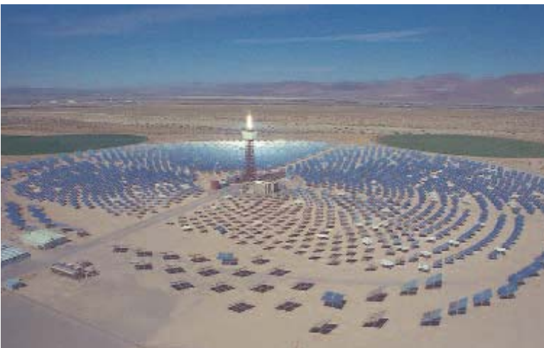
Solar tower power plant in Barstow, California
