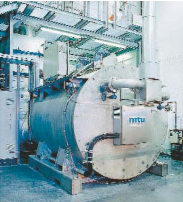
This fuel cell runs on natural gas. Hydrogen is produced in the unit and then converted to electricity and heat in the cells. A similar system is currently being equipped to run on biogas.
