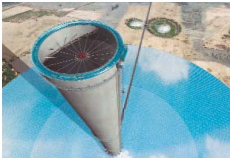
Tower of the planned 200-WM solar chimney power plant (height 1,000 m, with special spoked wheels for support), Below: the collector roof (diameter 6 km)
