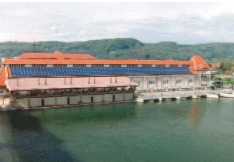
Photo caption: The renewable twin-power plant in Grenzach-Wyhlen uses hydropower and solar energy to generate electricity; bottom: Water steps at the hydroelectric power station Einsal an der Lenne
