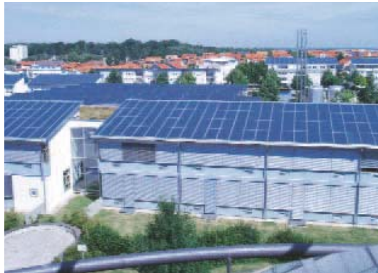
A large solar collector field supplies a local heating grid in Neckarsulm.
