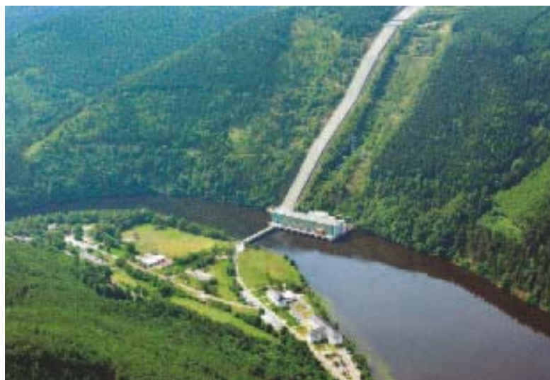
Pumped-storage power station Hohenwarte an der Saale
