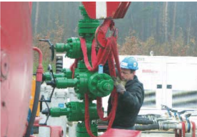
Capping a bore hole and preparing for hydraulic tests
