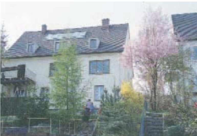
Collector system for domestic hot water
