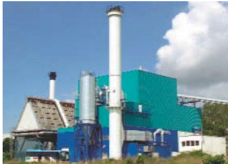
Biomass cogeneration plant in Demmin
