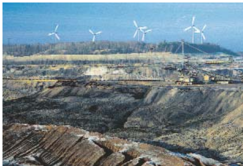
In Klettwitz (Brandenburg) one of the largest European windparks (38 turbines) was built on the top of mining waste heaps.
