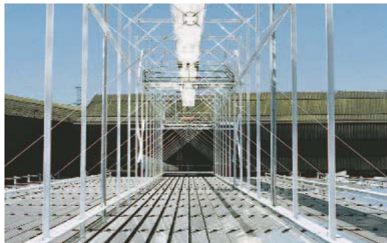
Collector system of a Fresnel system. Below: the mirror sections of the Fresnel reflector, Above: the absorber pipe at the centre of the secondary-stage concentrator. One collector branch is 24 m wide and can be as long as 1 km in the power plant version.
