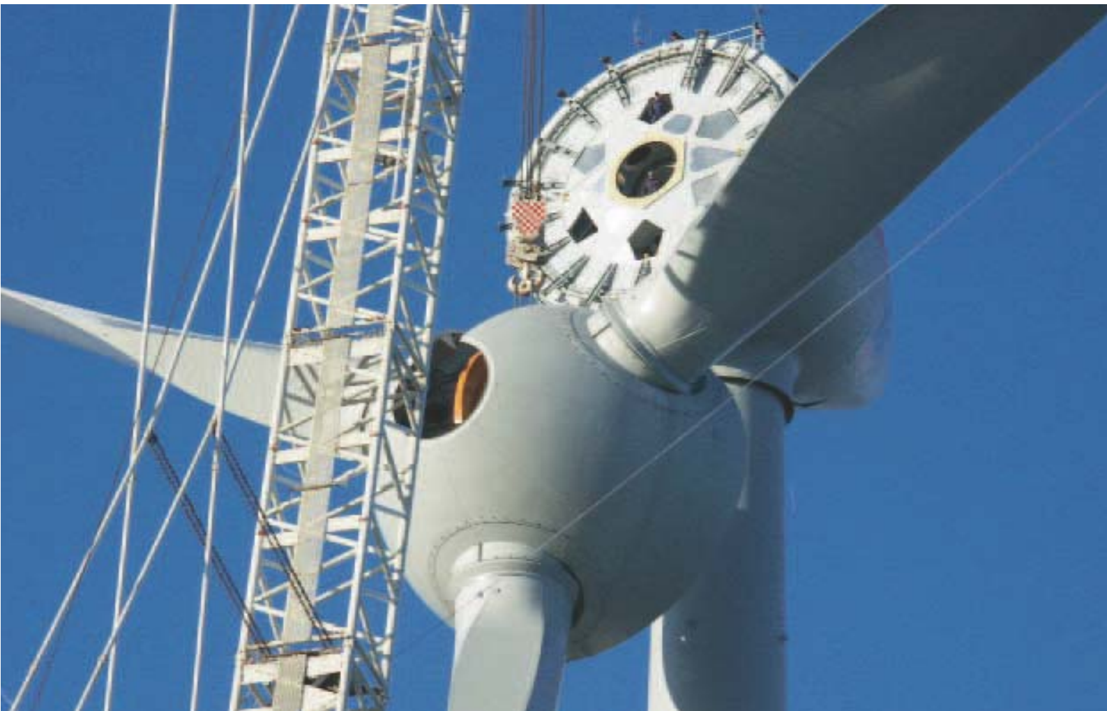
Assembly of a 6-MW wind power station
