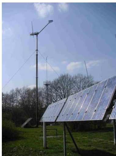
Fig. In the Garden of Energielabor
